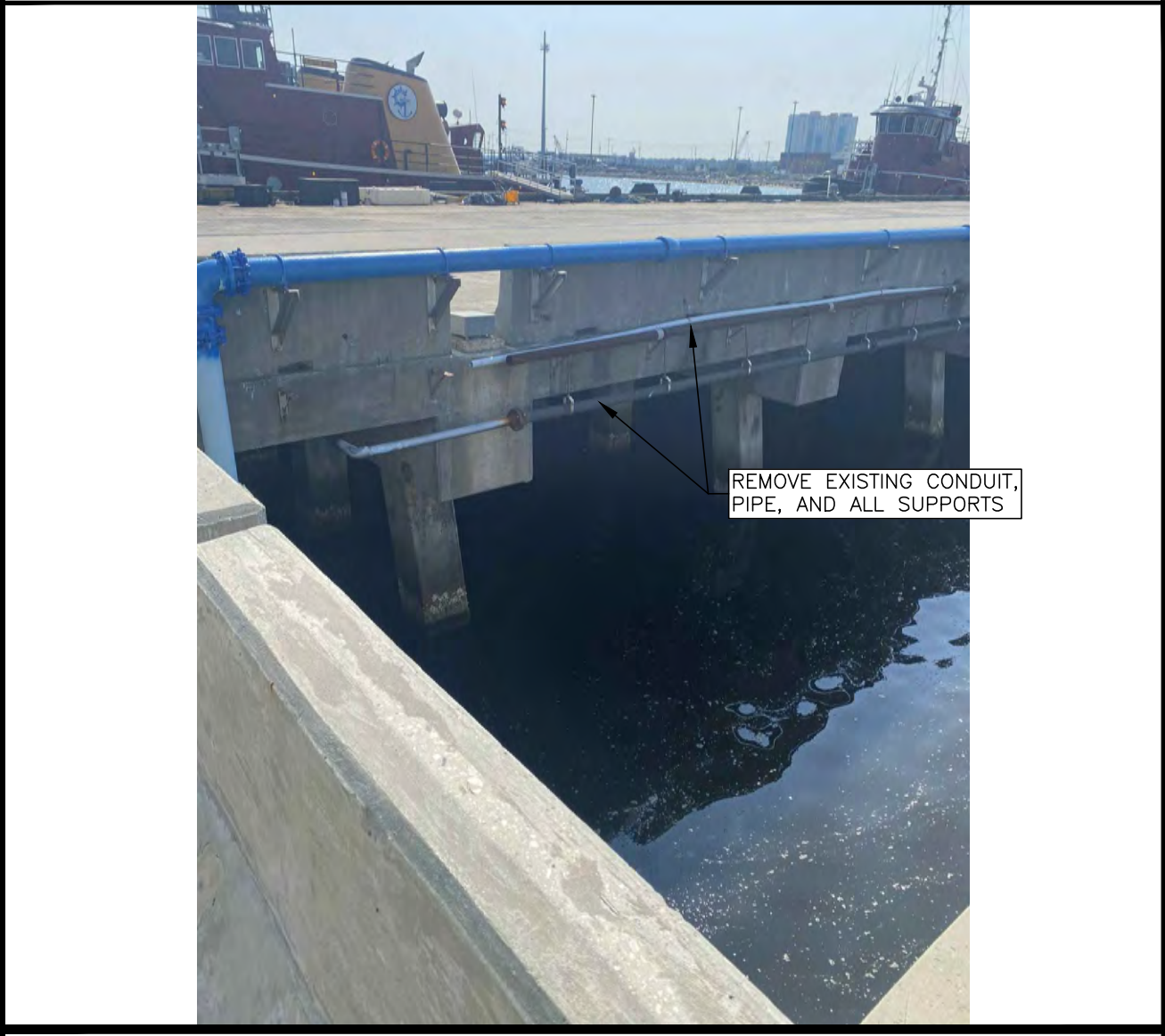
PIC #3 - EAST PIER DEMO
