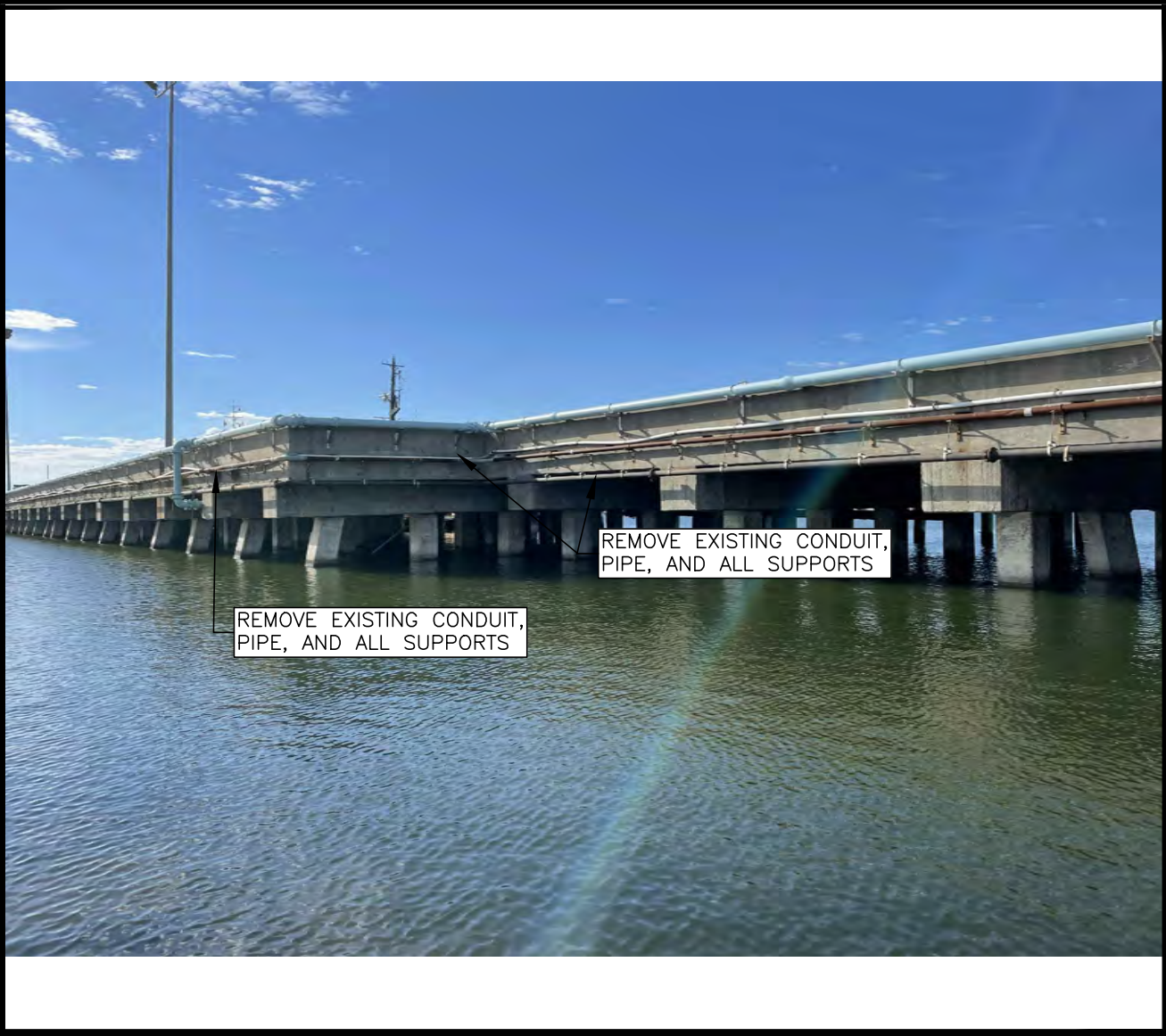
PIC #4 - EAST PIER DEMO
